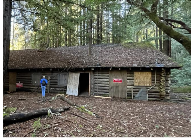
Figure 8. Close-up of south end of west façade, facing southeast.
