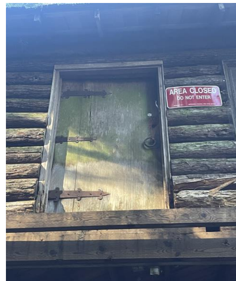
Figure 3. Detail of front entry door and ironwork.
