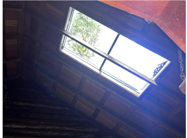
Figure 5. Typical aluminum skylight, as seen from the interior.
