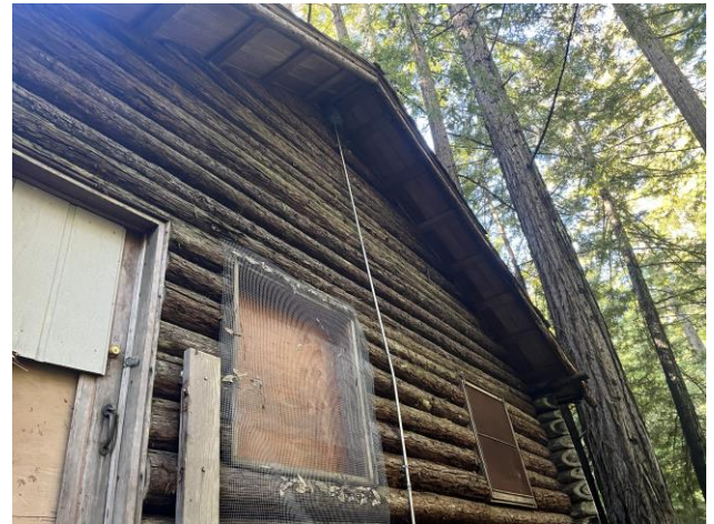
Figure 10. North façade entry door and windows.
