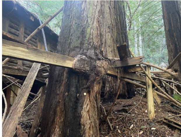
Figure 11. Remnants of rear porch projection at the northwest façade.
