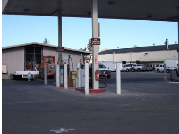
Project Site 2 – Site Photographs
