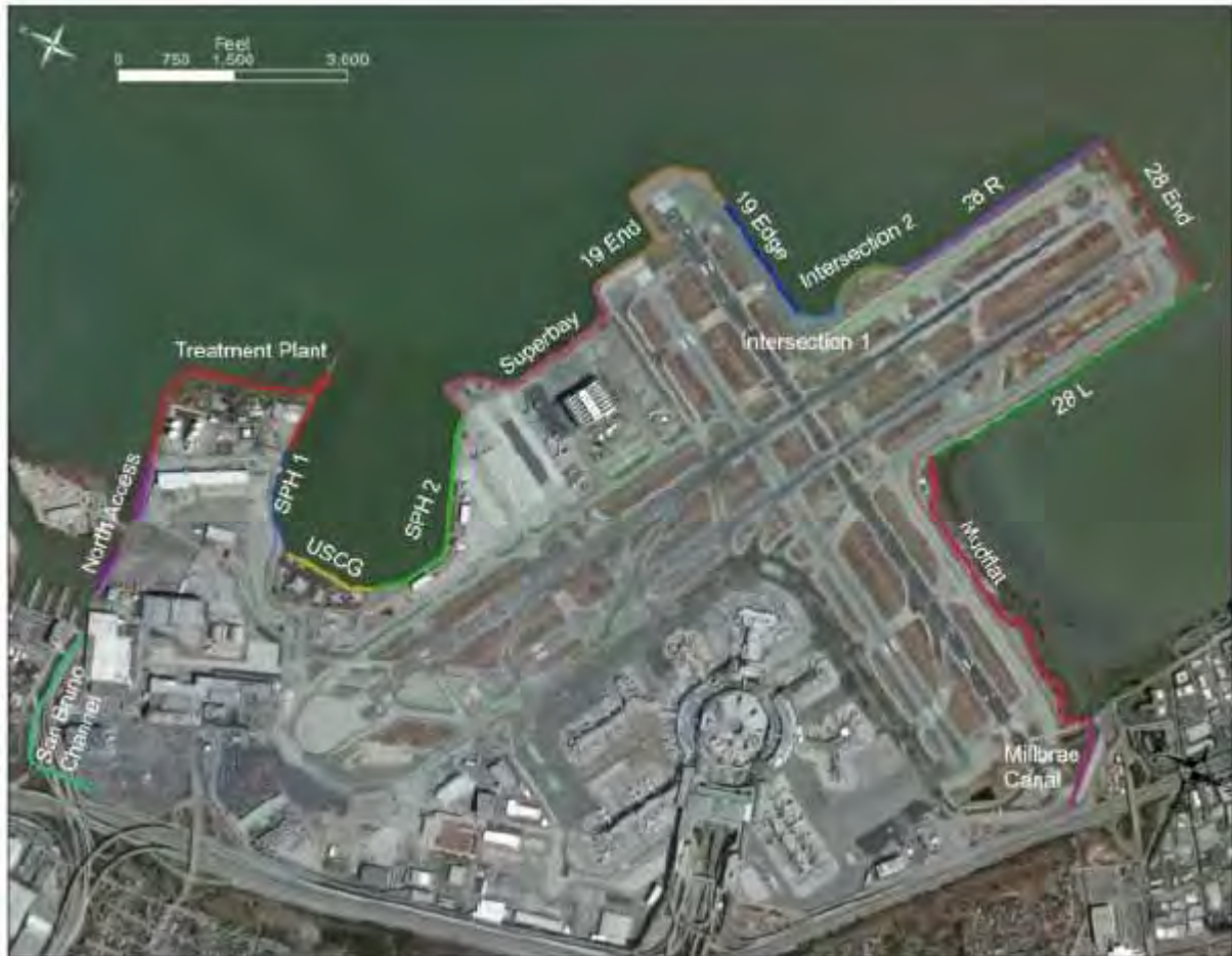
Figure 3-8: San Francisco Airport Shore Protection Structures
