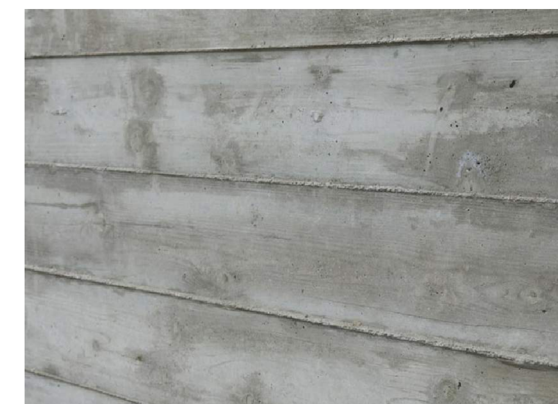
4 | BOARD FORMED CONCRETE NTS
